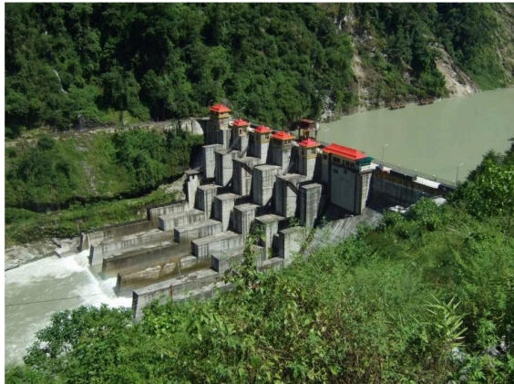
Fig : Teesta-V Hydropower Station
